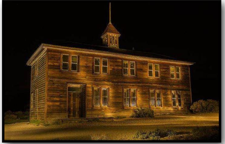
Fourth Place “Light Painted Old School House” by Jan Gemeinhardt
